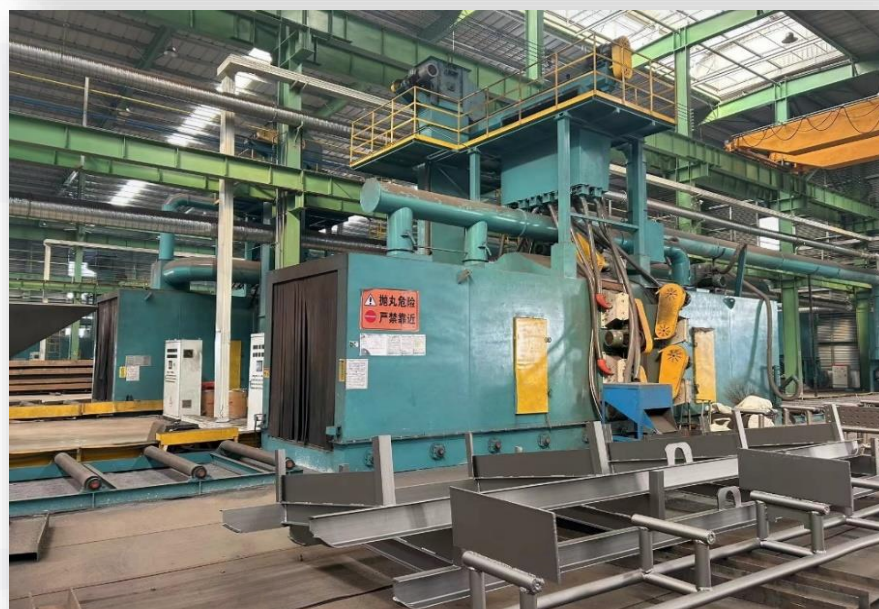
Sand blasting room
