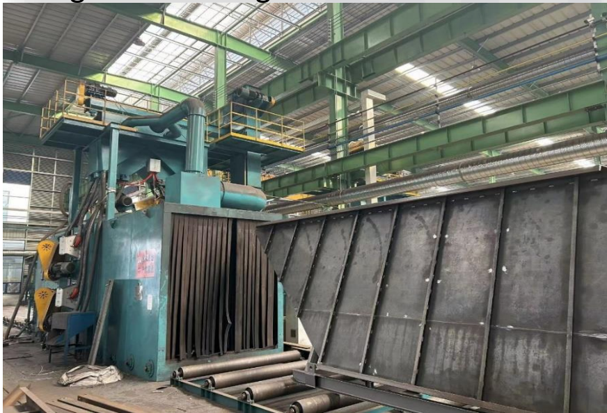
Sand blasting room
