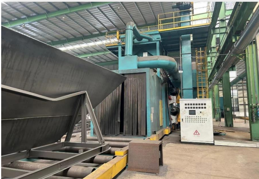
Sand blasting room
